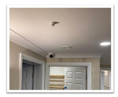
In the image above we can see the nozzle in-situ and also showing how the position of the head has been co-ordinated with other services (such as lighting plans and smoke detection) to provide compliant cover and not interfere with the overall look and feel of the interior design.
