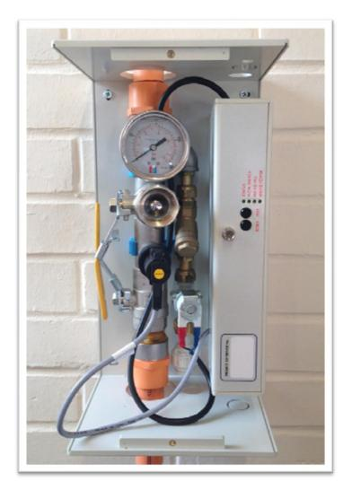
Our unique Automatic Testing & Control System (ATACS) constantly monitors the whole system. Designed to meet a specific requirement of the watermist British Standard (B.S.8458:2015) it carries out an automatic test on a rolling 28 day cycle.
