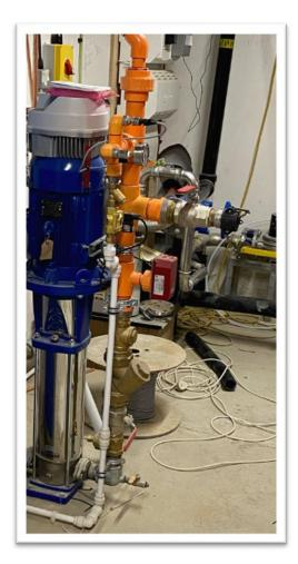
Working closely with our client, the fire suppression system water supply is shared with the domestic demand. There are advantages to this; cost, space-saving and a reduction in the time needed on site.
